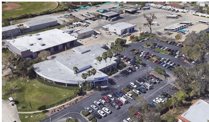
Figure 3-5: Votran Administration and Operations Facility
