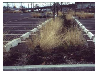
Stormwater Quality Swale in Parking Area, Portland, OR
